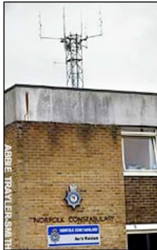
The mast at the North Walsham station
